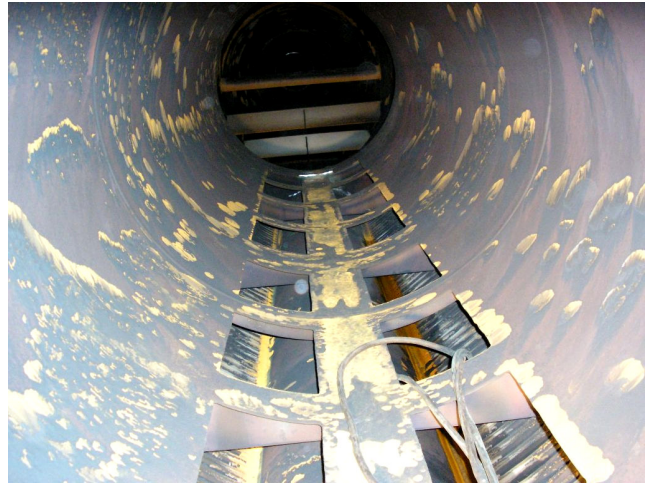
Photo 16: Upper distribution duct; DHACI rating 3 at tube inlets
