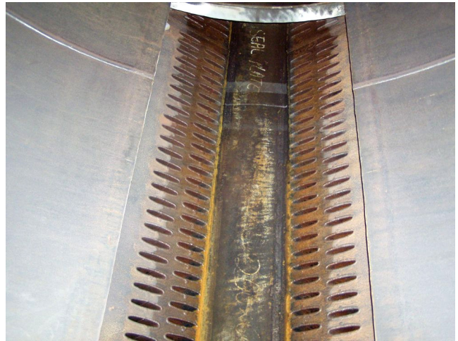
Photo 17: Tube inlets in upper duct; DHACI rating 1 at tube inlets
