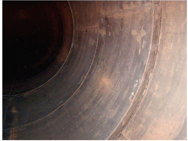
Photo 10: Lower duct DHACI rating A
