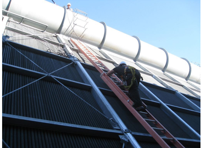
Photo 4: Upper duct with difficult access to manway on top side.
