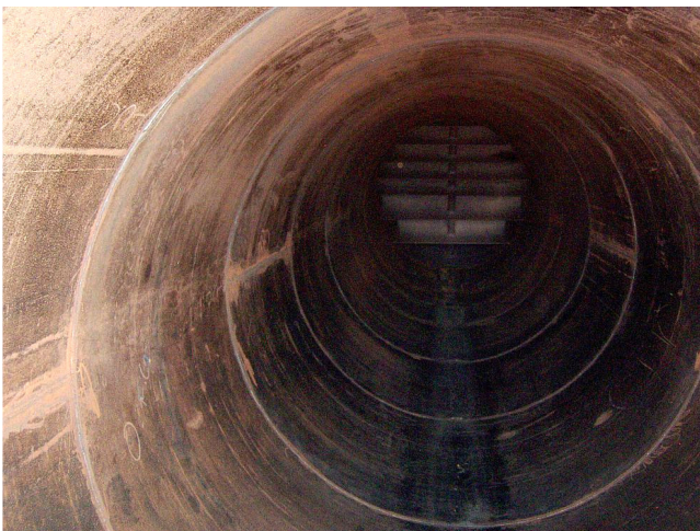
Photo 15: Lower distribution duct section, including risers
