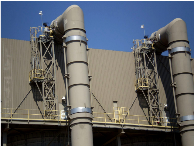
Photo 3: Permanent ladder access to upper duct, with permanent platforms at manways.
