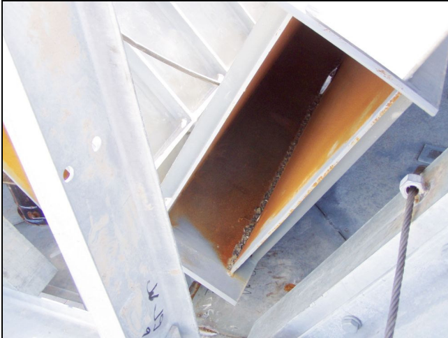
Photo 1: Debris in lower ACC header; weld flux containing high concentrations of fluorine.
